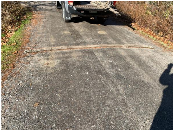
One of three speed control ropes in three-season use on this 900-foot private way for at least 10 years to general acclaim.
